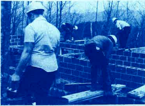
Beech Golf Course Clubhouse-Lounge Under Construction
